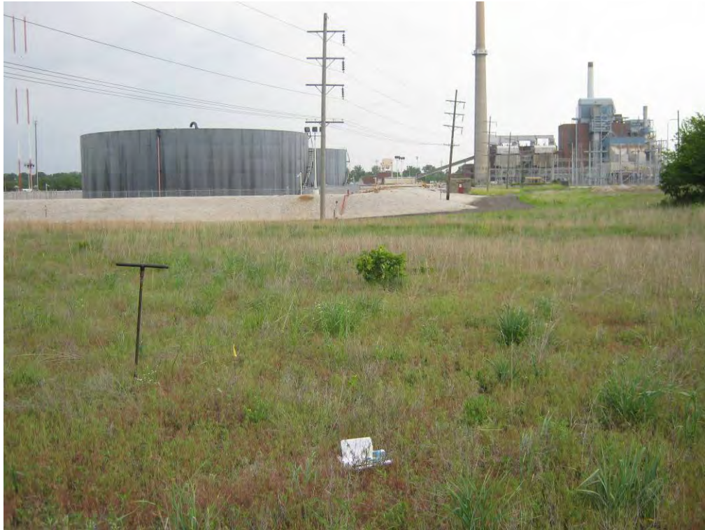
Photo 13. View looking northwest across a portion of Area 7 towards existing fuel oil storage tanks.
