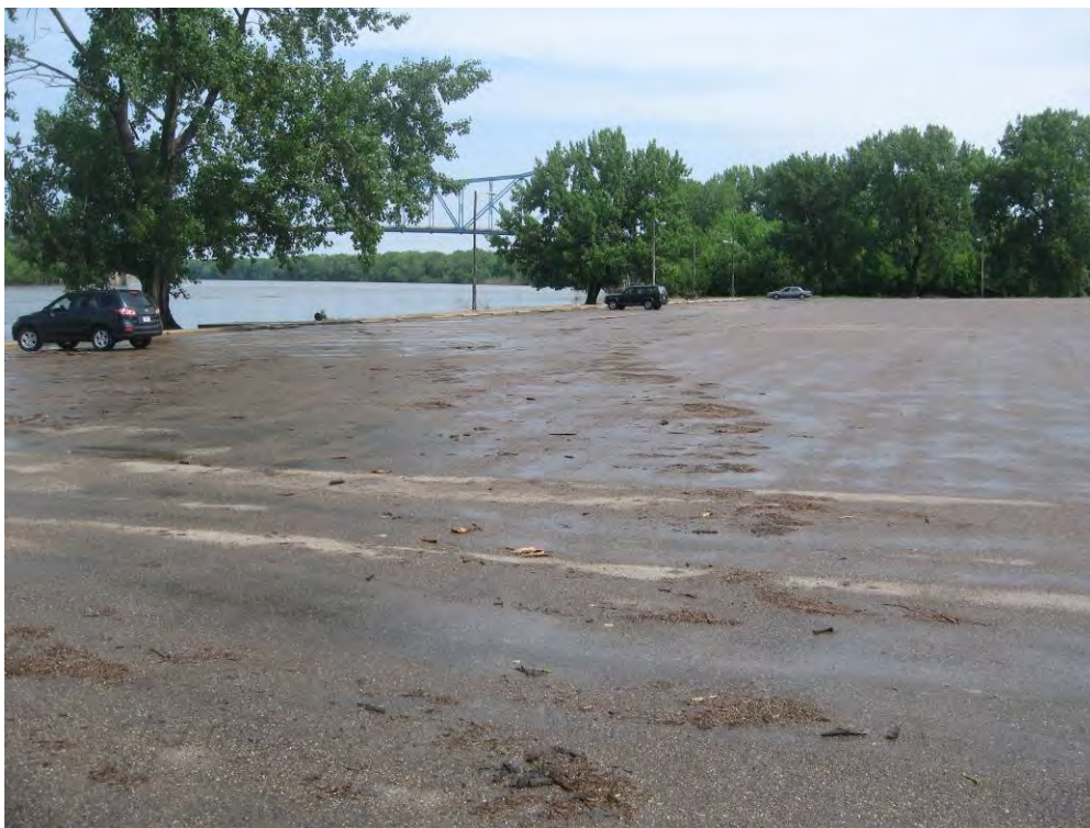
Photo 2. Edge of parking lot and beach adjacent to boat ramp on Village Property (Area 1).
