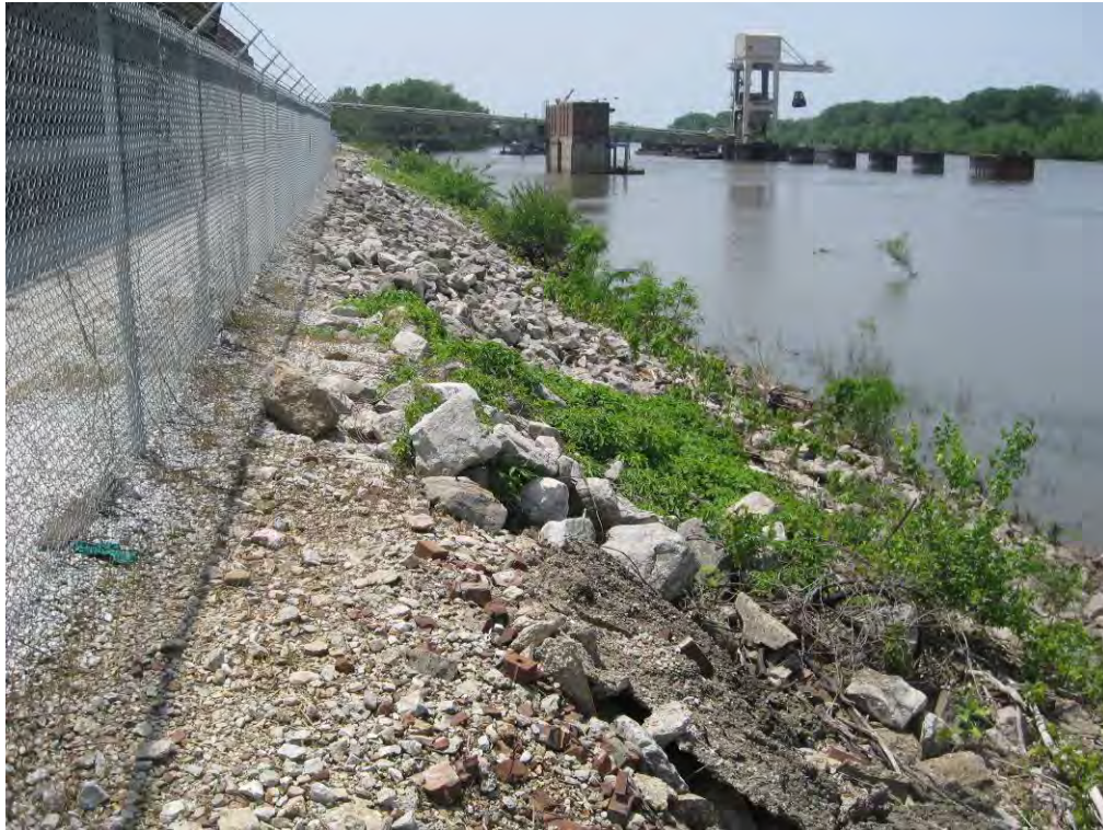
Photo 3. Existing rip-rap bank on west side of Ameren facility along the Illinois River.
